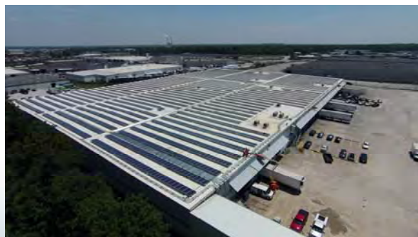
Grocers Supply Roof, 1MW rooftop system.
