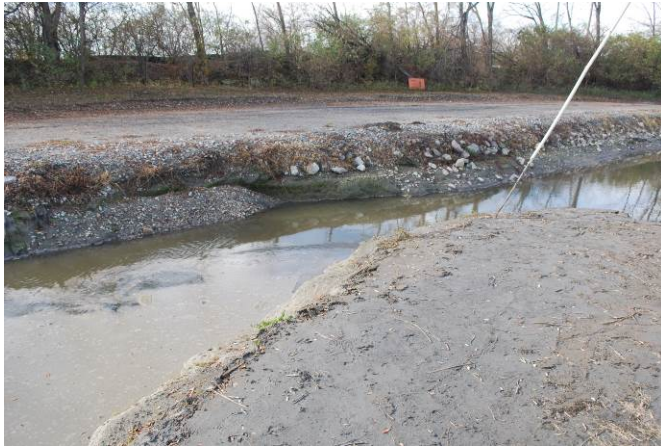
Photo 10: Breach excavated in the South abutment of the intermediate dike between former Pond 2A and Pond 2B. Some erosion of the interior slope in the abutment.
