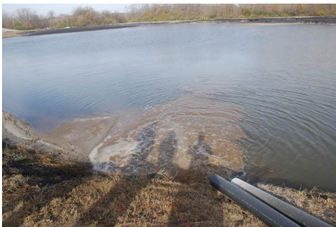
Photo 9: FGD slurry discharge into Pond 1.
