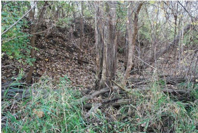
Photo 22: Conditions of the exterior slope of the North perimeter dike of Pond 3, looking west from the outfall structure. No seepage observed.
