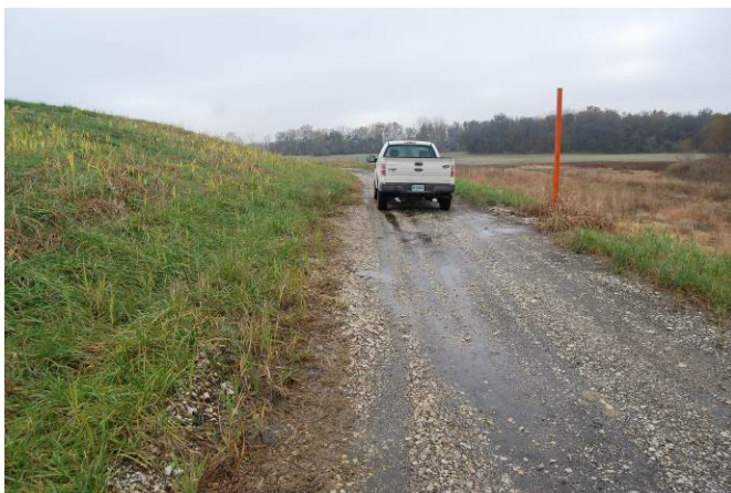
Photo 33: Fluid conditions at the toe of the upper dike of the northeast corner of Pond C. Heavy rainfall occurred in the days prior to the inspection. No active visual seepage occurring at the time of the inspection. Looking west.
