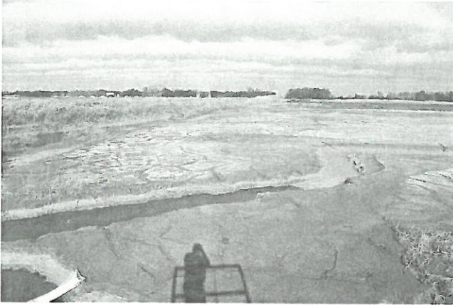
Photo 28: Pond C, looking west from discharge box of Pond C.
